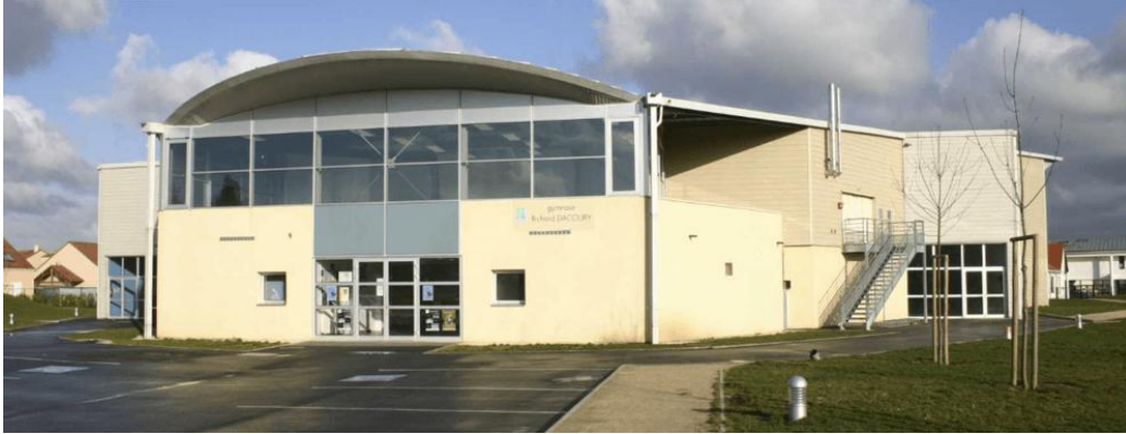
Gymnase Richard Dacoury – Source : GPSSES
